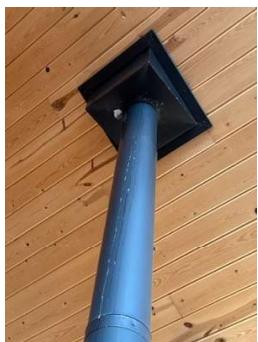
**Connection to Factory-Built Chimney/Vent:** Improper ceiling support box installation, Other Issue
