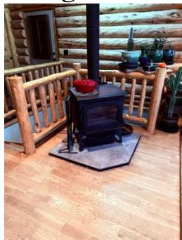
**Base appliance:** Hearth/Heating, **Base hearth / heating:** Stove, **Base appliance fuel:** Wood, **Brand:** Timberwolf, **Model:** 2200, **Serial #** EPA2020 007929, **Mfg Date/Code:** Nov 2010, **Flue Collar Outlet Diameter:** 6", **The BASE appliance is connected to the following type of chimney/vent:** Factory-Built, **Height/Length of Flue/Vent in Feet:** 18',
