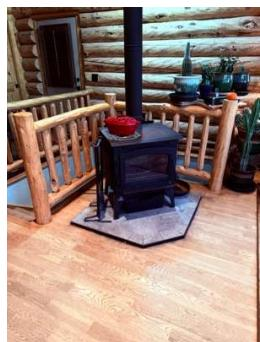
**Base appliance:** Hearth/Heating, **Base hearth/heating:** Stove, **The base system was** Inspected, Swept, Internal Camera Inspection Performed
