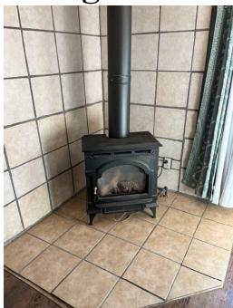
**Base appliance:** Hearth/Heating, **Base hearth / heating:** Stove, **Base appliance fuel:** Gas (Natural), **Brand:** Vermont Castings, **Model:** OXDV30NV, **Serial #** OXDV30NVB1204000001, **Mfg Date/Code:** -, **Flue Collar Outlet Diameter:** 4", **BTU**
