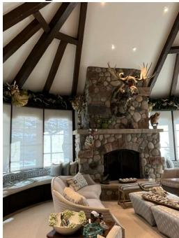
**Base appliance:** Fireplace, **Base fireplace:** Masonry Firebox (Site-Built), **The BASE appliance is connected to the following type of chimney/vent:** Masonry, **Height/Length of Flue/Vent in Feet:** 24,
