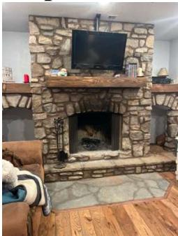
**Base appliance:** Fireplace, **Base fireplace:** Factory-Built Fireplace, **Base appliance fuel:** Wood, **Brand:** Hearth & Home, **Model:** EXCLAIM-36, **Serial #** C5 1639981, **Mfg Date/Code:** 12/01/2021, **The BASE appliance is connected to the following type of chimney/vent:** Factory-Built, **Height/Length of Flue/Vent in Feet:** 18, **Explain offsets, their angles, and location within the system?** 2 45s after one small section off the base of the unit
