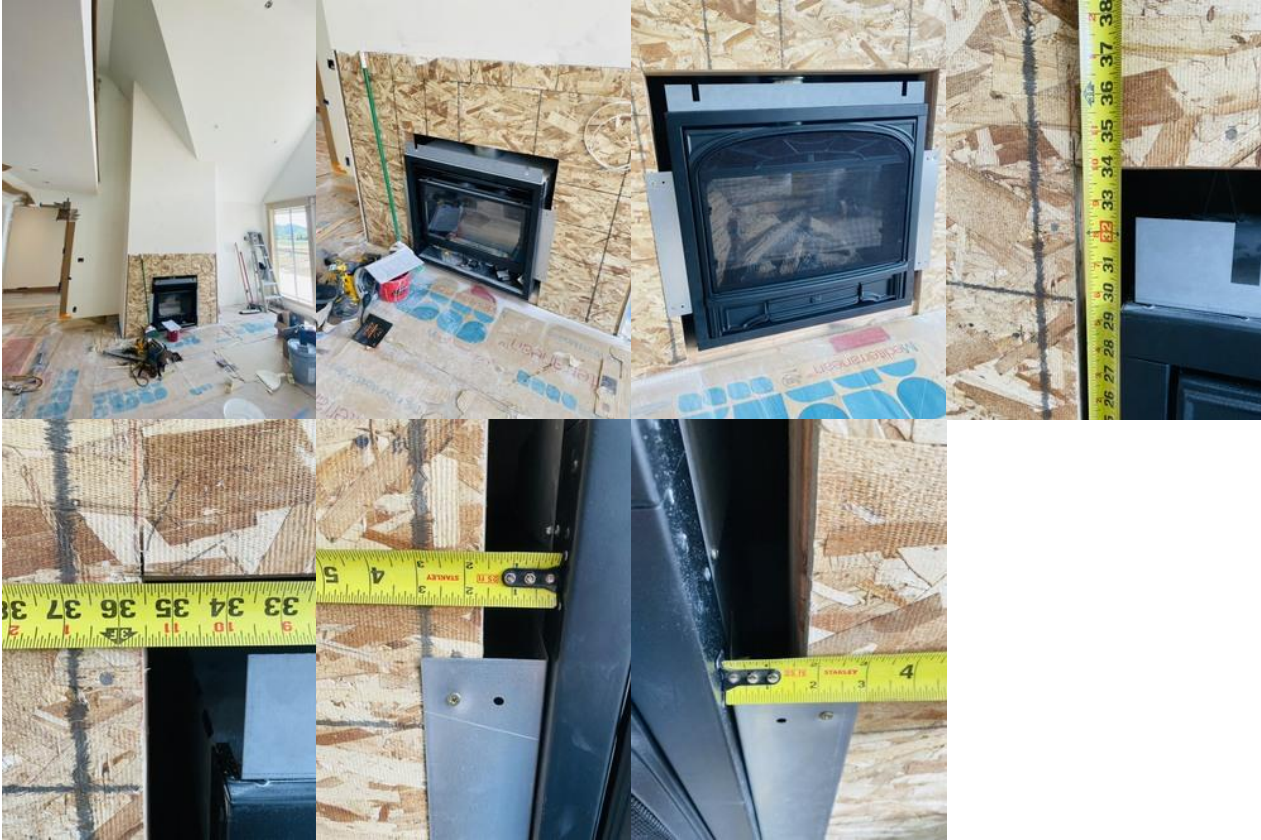
Unit upon arrival, following adjustment for tile finishing, measurements and clearances.
